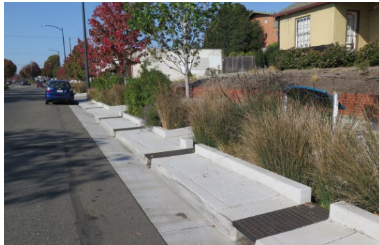
Permeable paving treatment
