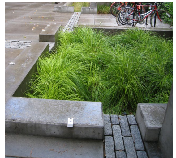
Roof downspouts drain to planting area
