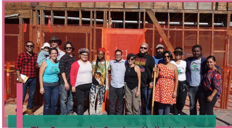
The Community Services Unlimited team at the groundbreaking of the Paul Robeson Community Wellness Center.
